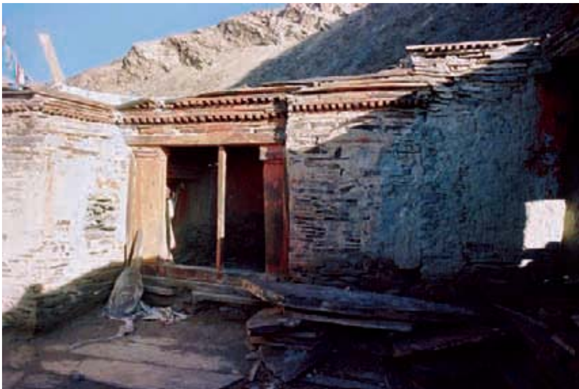
Fig. 370. The inner courtyard of Ri'u dgon-pa (B-25)
