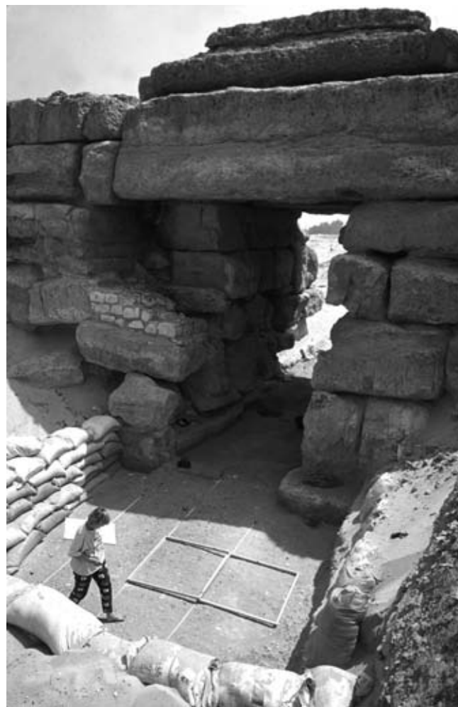
Fig. 5 The north side of the gate through the Wall of the Crow, cleared in 2001. View to the SE
