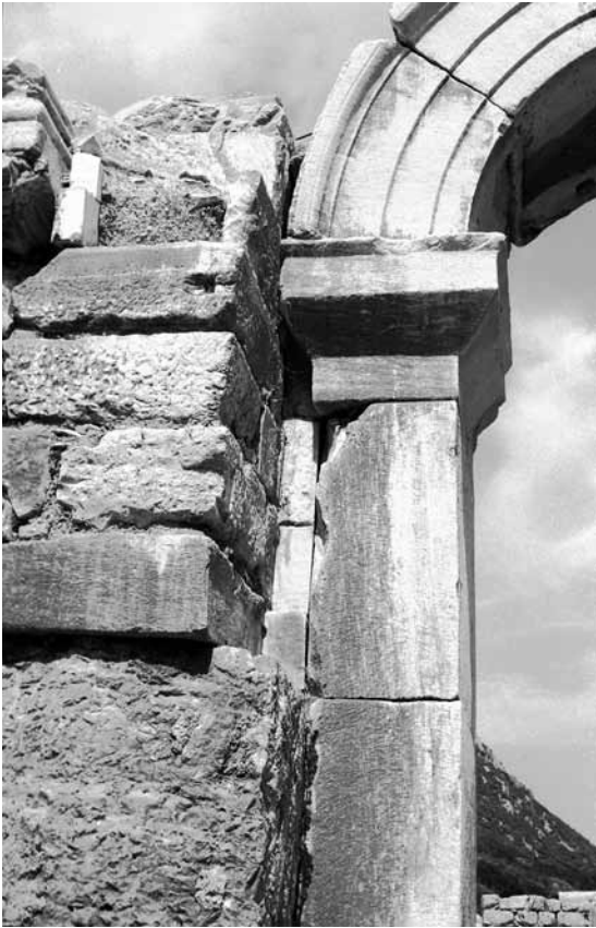
1 South jamb of western arched doorway from east
