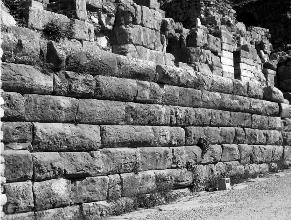
1 Masonry of the scaenae frons of the Great Theater in Ephesos
