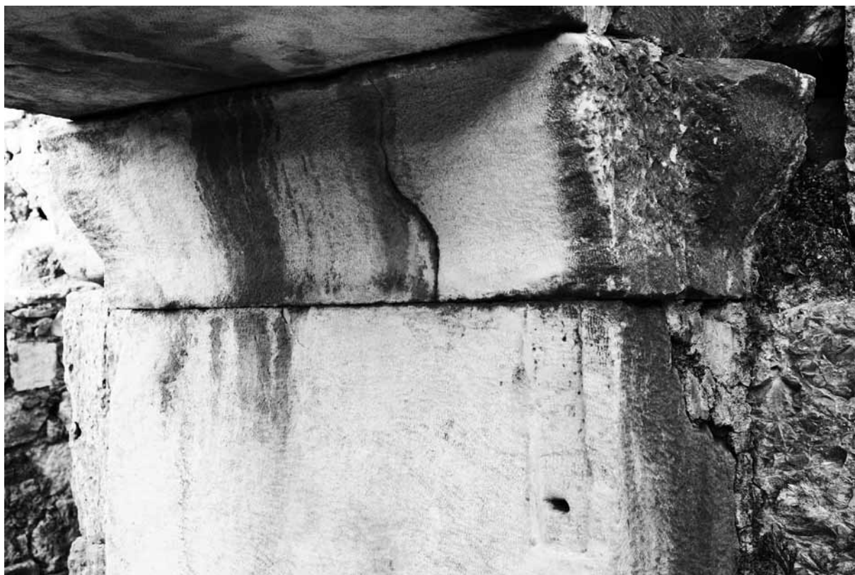
3 West parodos , SD 1: cutting in eastern door jamb
