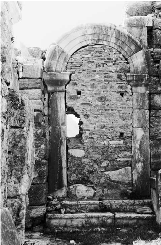
2 Blockage of western doorway between Bouleuterion and Rhodian Peristyle
