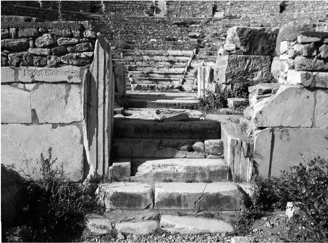
1 Central door through Basilica Stoa (BD 3), north wall, with Bouleuterion SD 4 behind
