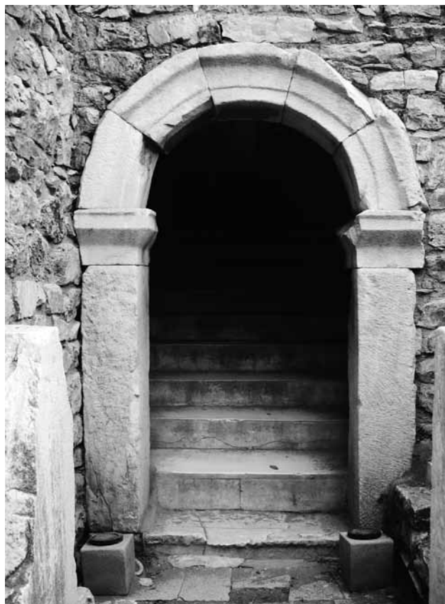
3 Access to the vomitorium staircase from the west parodos
