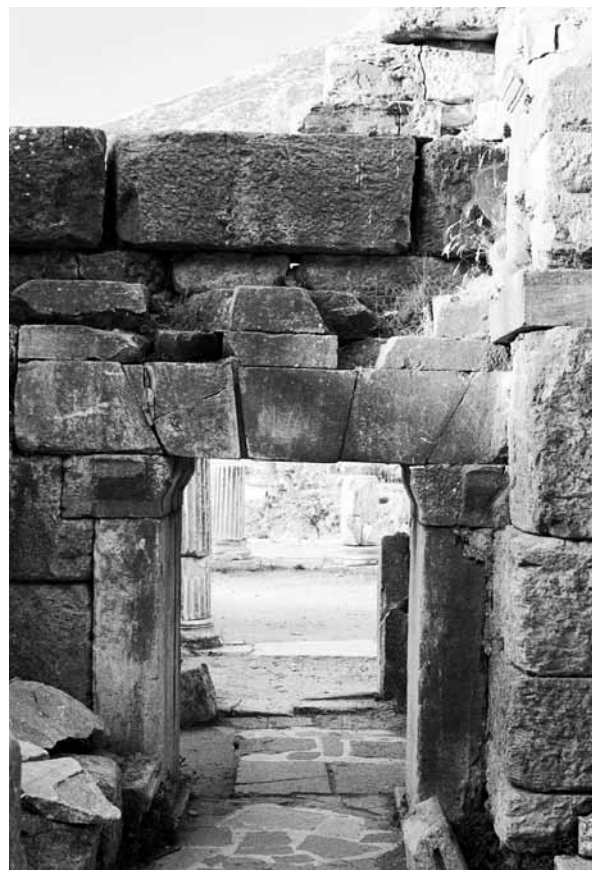
2 Doorway in west parodos from north (SD 1)
