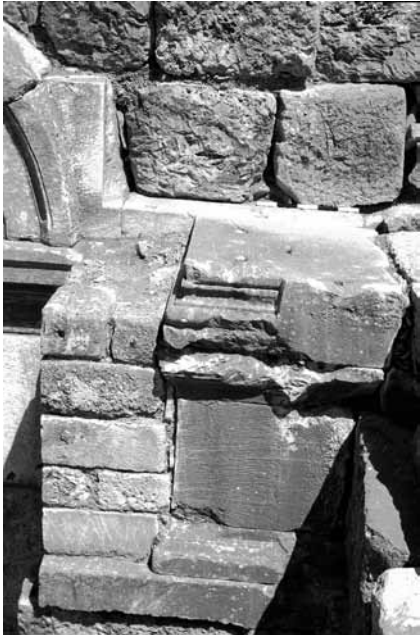
2 Pedestal and base in south-east corner
