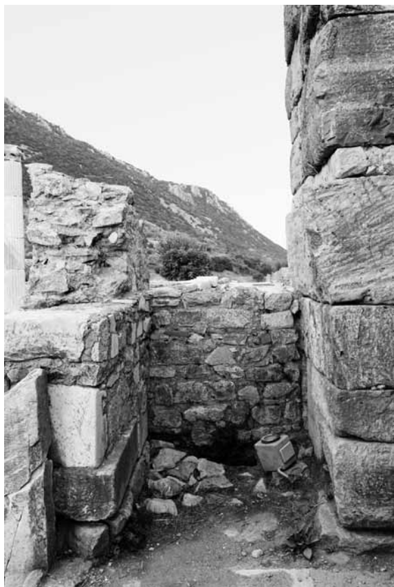
1 Short wall between west pier and Basilica Stoa
