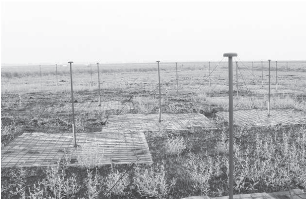
Figure 2: A part of a LOFAR LBA field. The antennas are the thin wires stretching downward from the vertical plastic support rod to the ground plane below. Each station comprises 96 dual-polarised elements. Picture by ASTRON.
