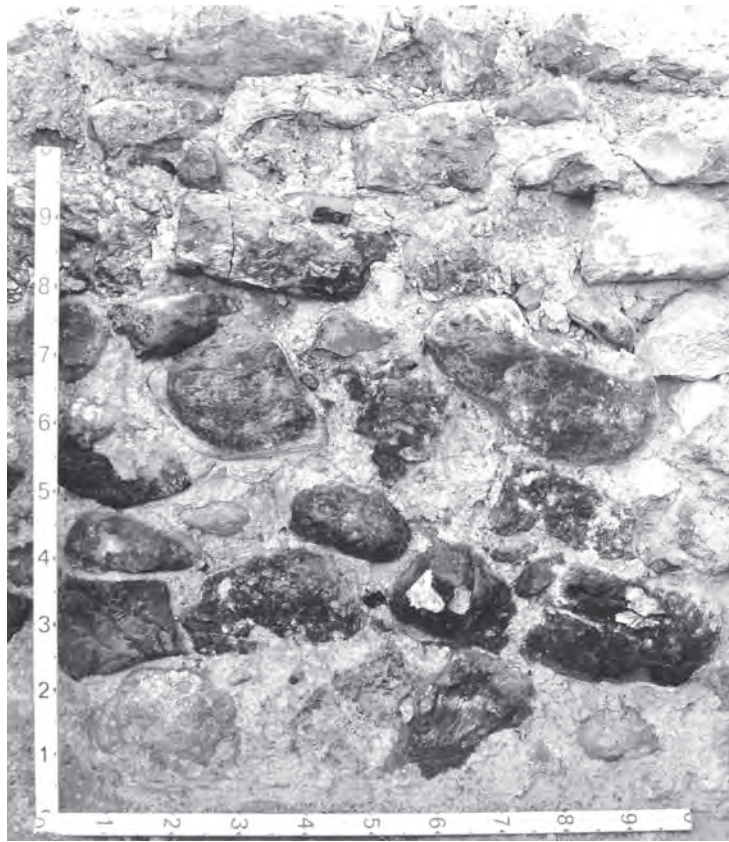
Fig. 252 Soot on northern wall of Room 19
