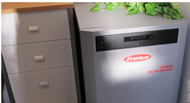
Battery for local storage of solar power in a private home
