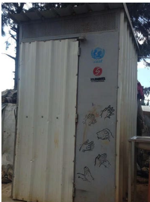
UNICEF's and Solidarités International's logos on the toilet of an informal tented settlement (one for more than a hundred people) in Akkar hamlet. March 2019.
