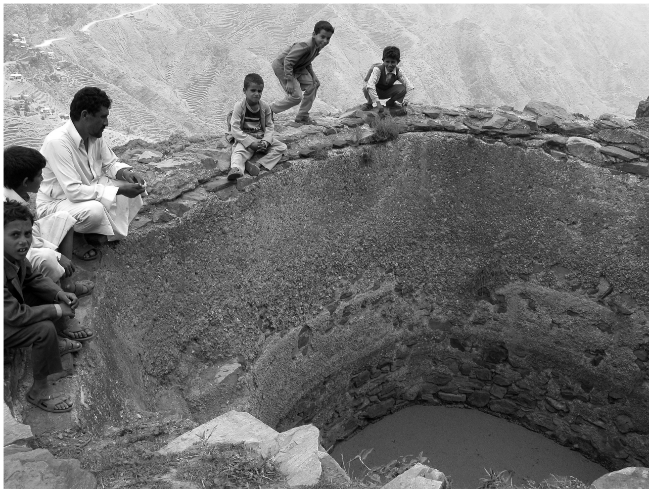
Figure 3: This is an old cistern where one can easily see how the qaḍāḍ has worn away near the bottom. The cistern was leaking and in need of re-plastering. (Photo: E. Hovden)
