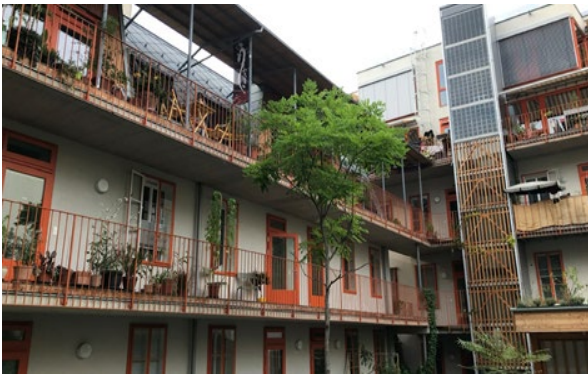
Multi-energy system, Geblergasse, 1170 Vienna
